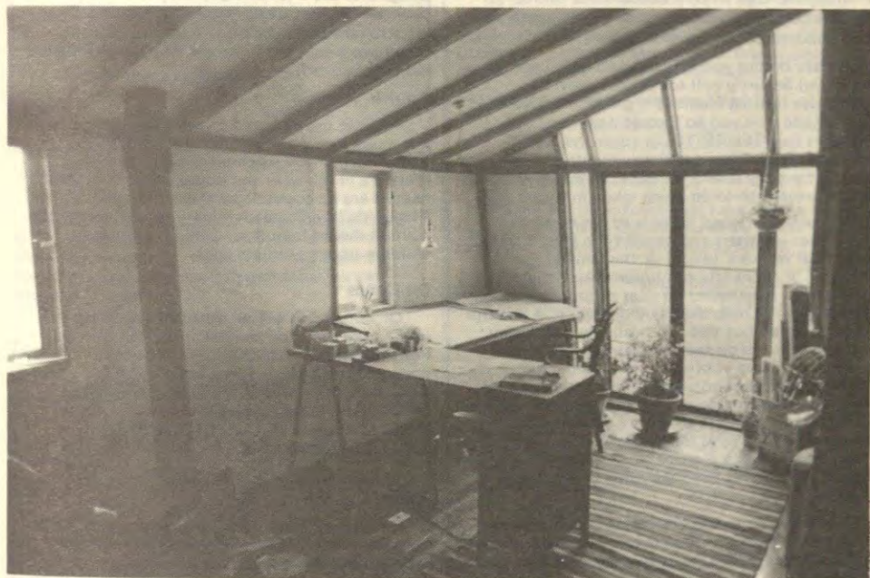
Extension built onto squatted house
