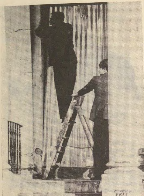
Removing corrugated iron
